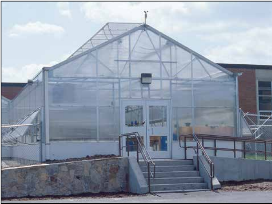
Upper Cape Cod Tech | Bourne, MA
