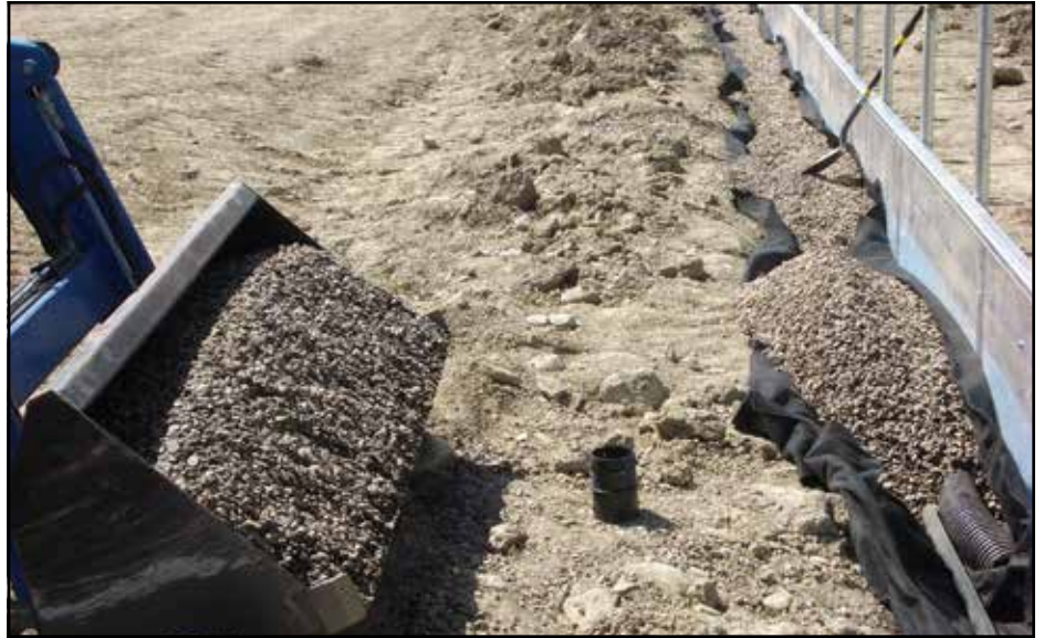
Good drainage is worth the investment.
