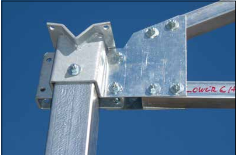
This photo shows how our truss is connected to our 4" column with a heavy duty saddle.
