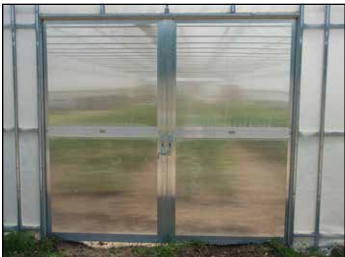
Double sliding doors with polycarbonate panels.
