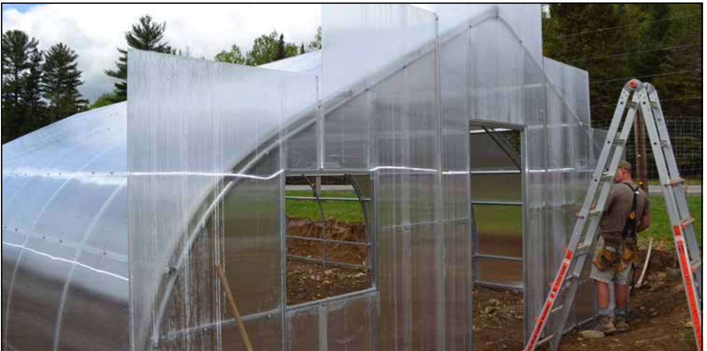
Polycarbonate installation on an end wall.
