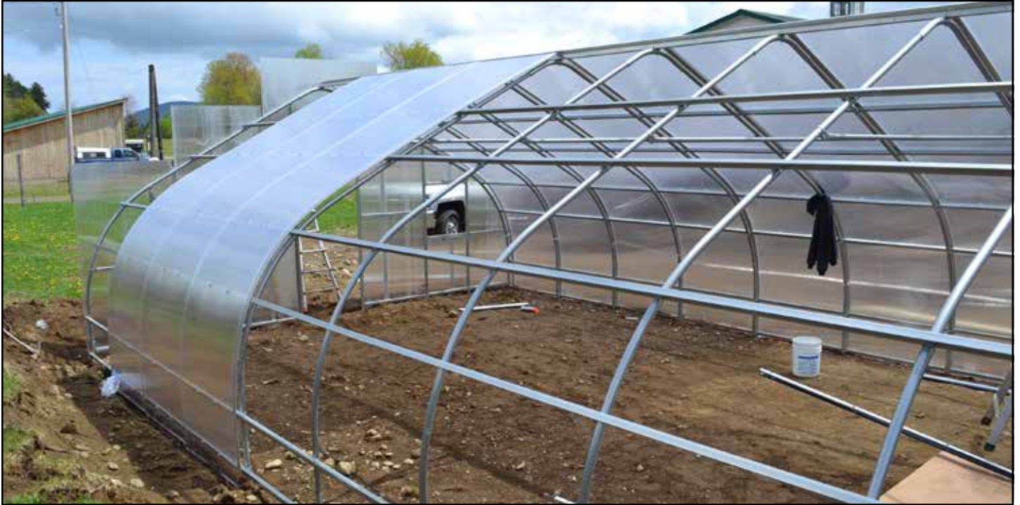
Polycarbonate installation on a roof.
