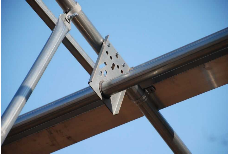
Shaft hanger on opposite side bow than the vent brace with 3 TEK screws Figure 8.3
