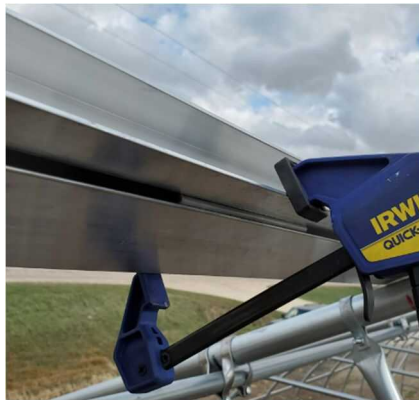
Maintain 1" gap between vent bottom rail and rail header Figure 4.0
